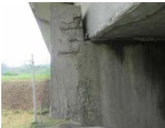
盖梁露筋锈蚀
