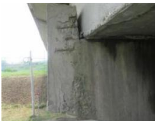
盖梁露筋锈蚀
